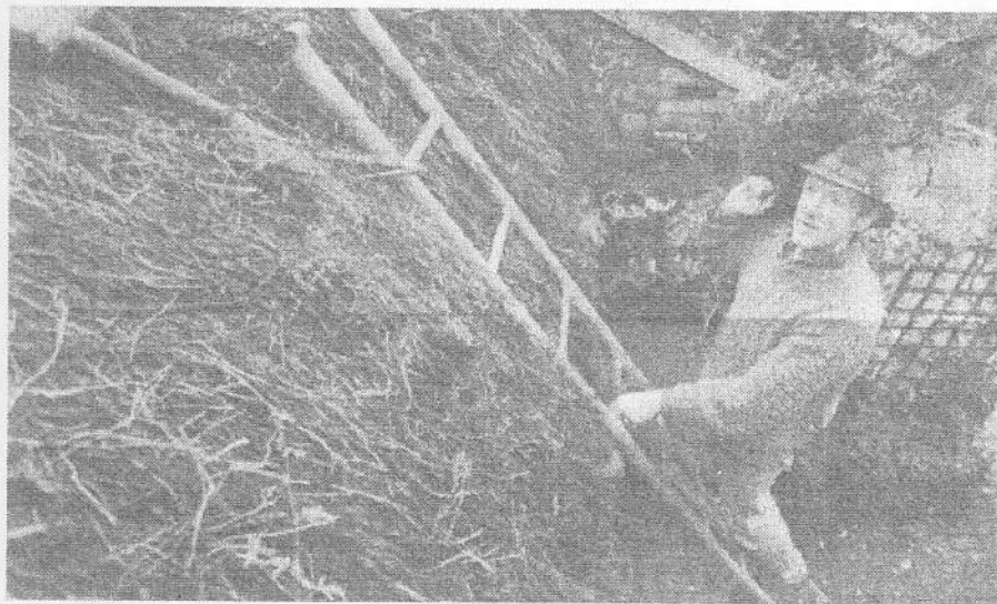
Durable: William Tegetmeier uses heather to thatch the roof of a cabin in York city centre. The master thatcher says the plant is in plentiful supply.
